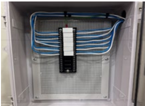
Inspect the Operating Status of SPDs
