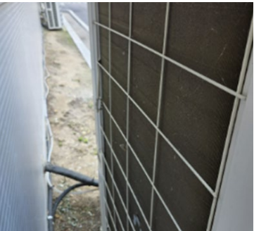
Outdoor Unit Fire Prevention Inspection
