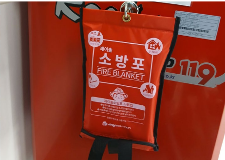
Lithium Battery Fire Extinguisher and Fire Blanket
